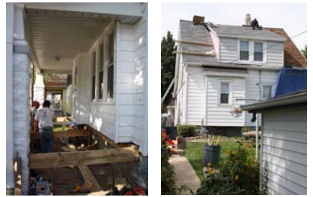
Harambee home under construction
